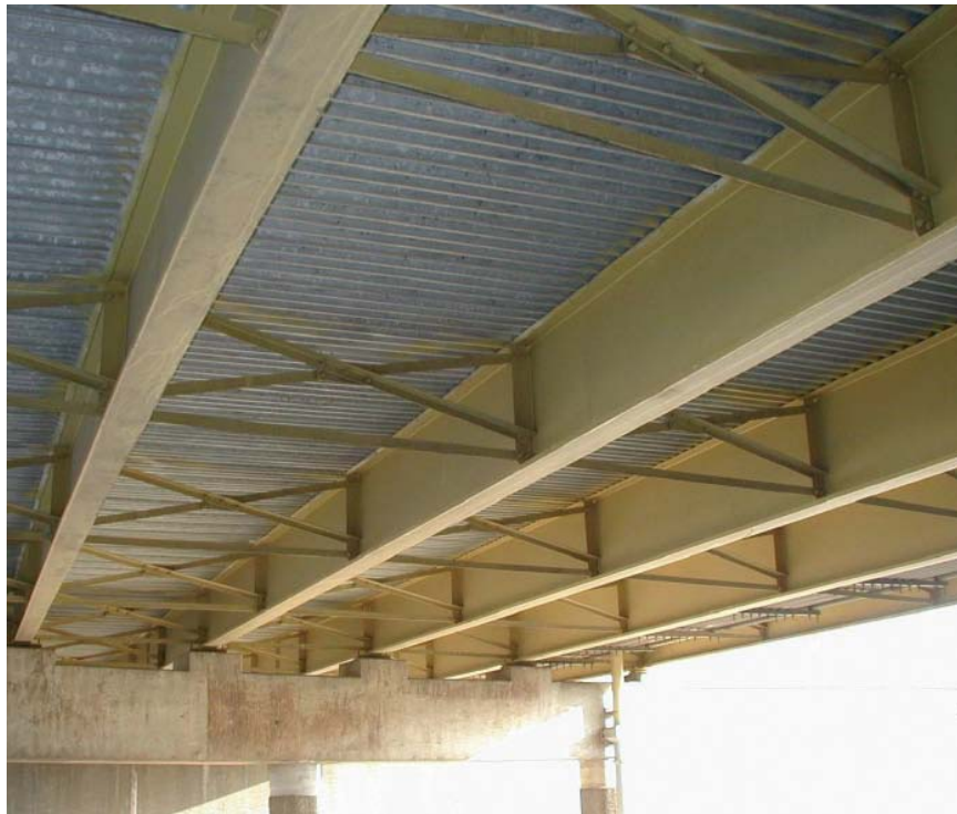
Figure 4-23 Steel Plate Girders as Bridge Superstructure [11]
