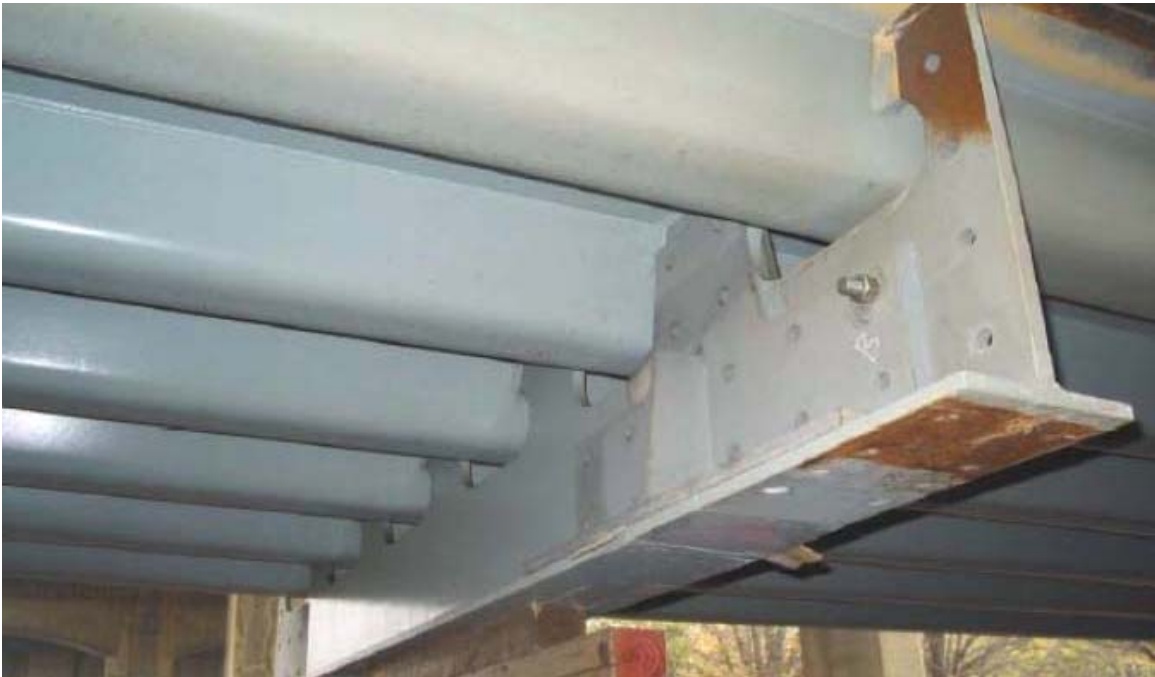
Figure 4-35 Underside of Steel Orthotropic Deck [25]
