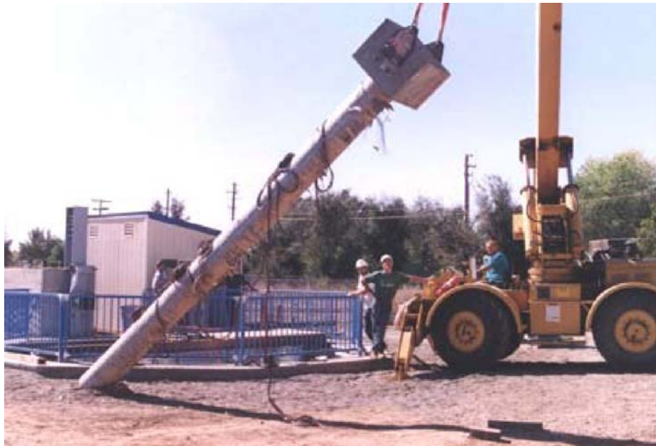
Figure 4-11 Precast Concrete Pile [39]
