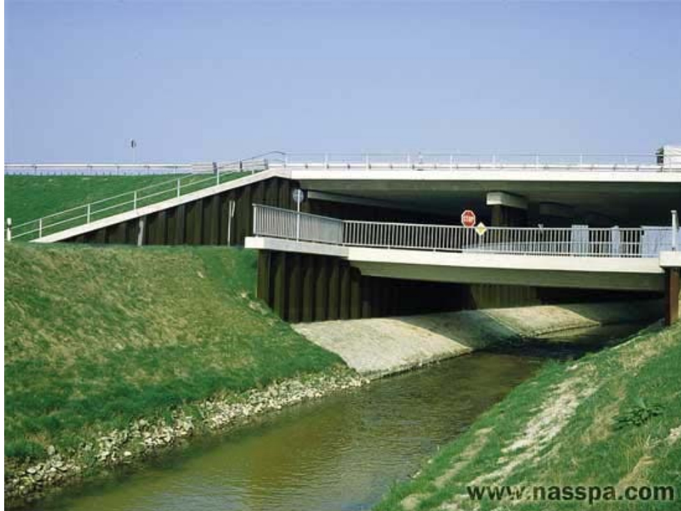
Figure 4-16 Steel Sheet Pile Wall Abutment [36]
