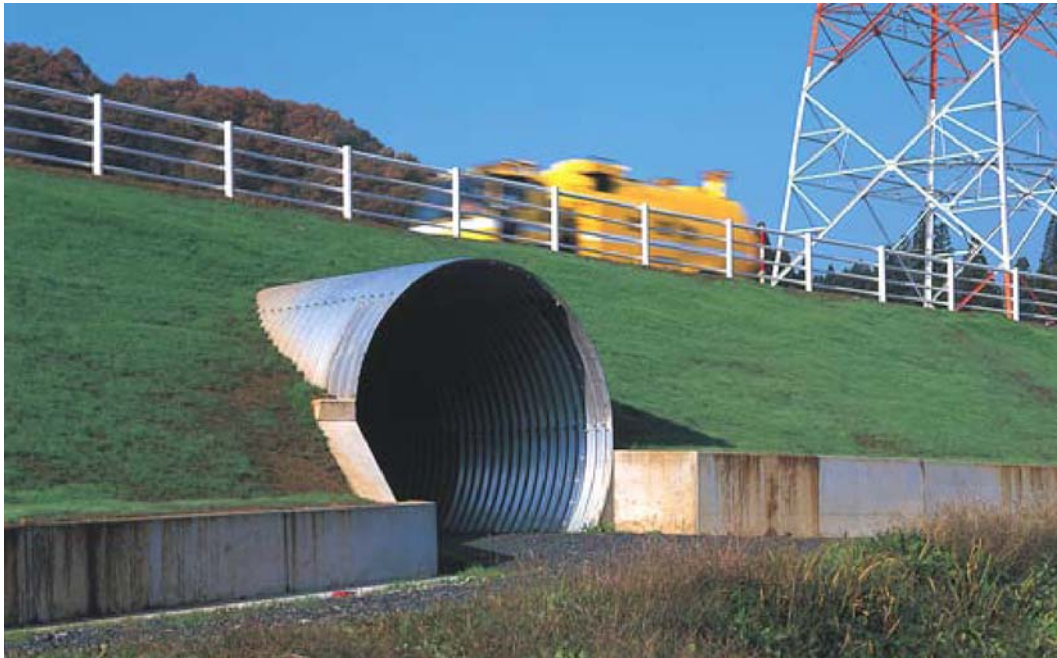
Figure 4-19 Corrugated Steel Pipe for Bridge Superstructure [15]
