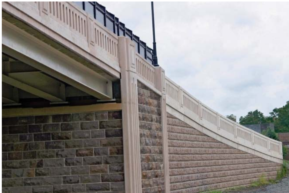
Figure 4-8 T-WALL® Wall System Installation [33]
