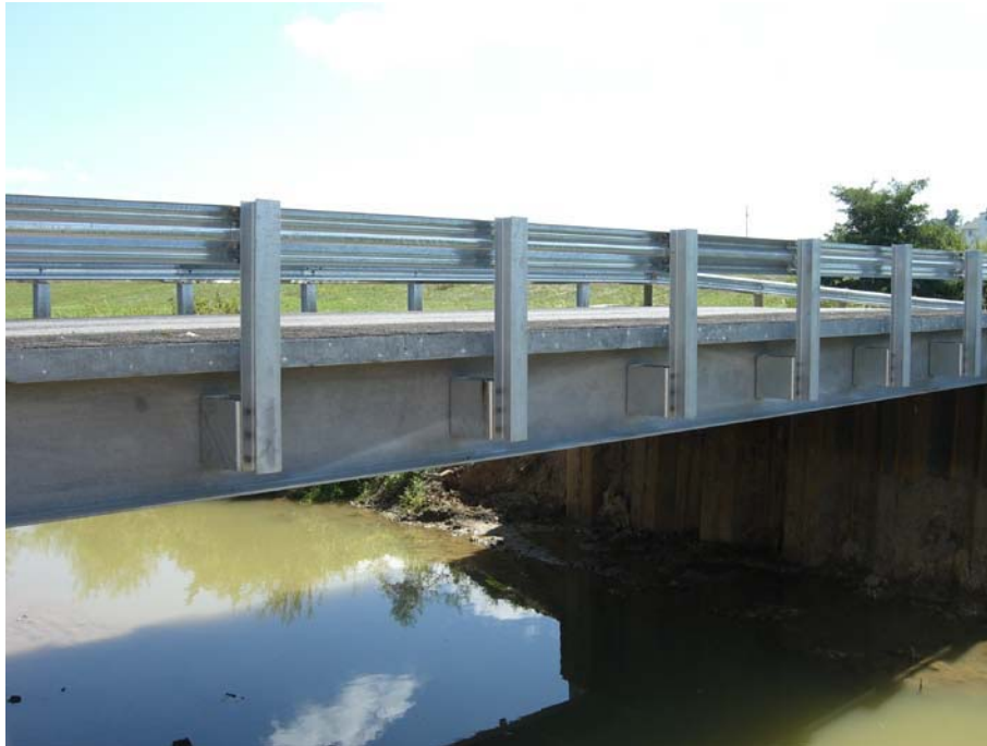
Figure 4-53 Steel Beam Rail Barrier (U.S. Bridge Tour)
