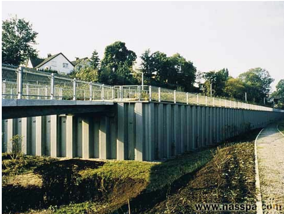
Figure 4-17 Steel Sheet Pile Wall Abutment [35]
