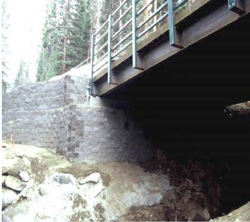
Figure 4-7 Geosynthetically Confined Soil Bridge Abutment [18]
