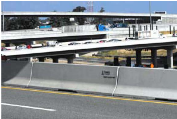
Figure 4-55 Precast Concrete Bridge Barrier [49]
