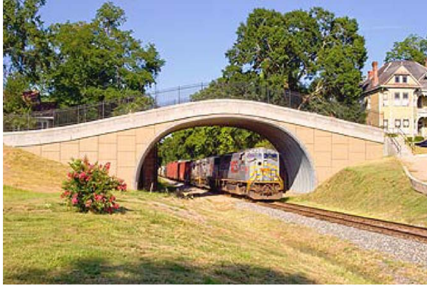
Figure 4-20 Corrugated Structural Plate as a Bridge Superstructure [9]
