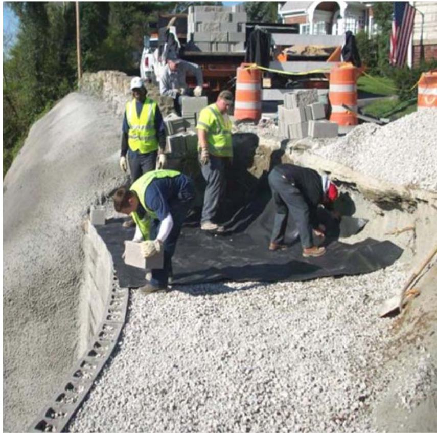
Figure 4-6 Installation of Geosynthetically Confined Soil Wall [19]
