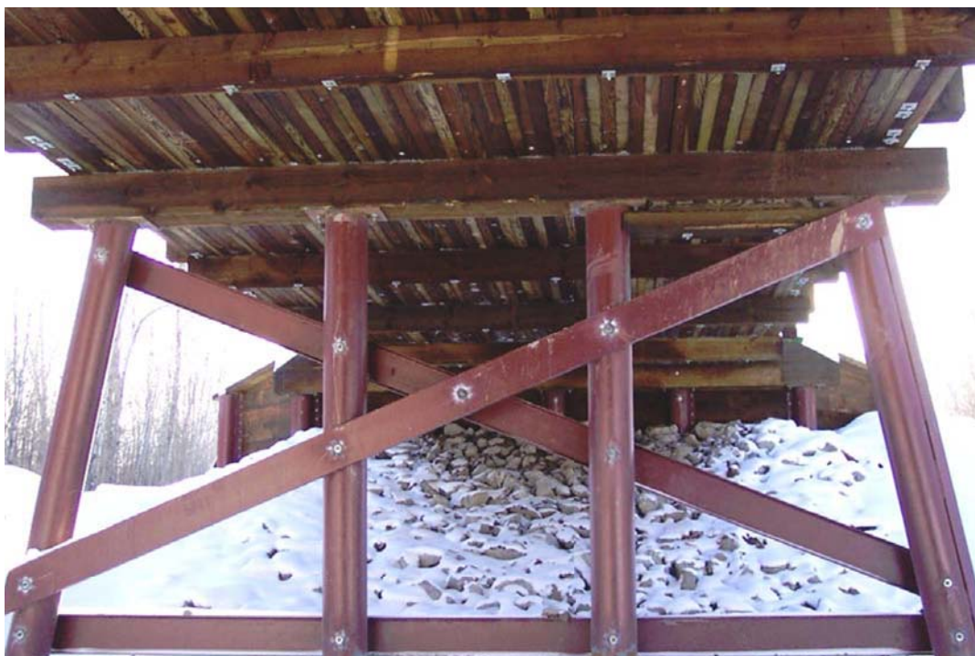
Figure 4-13 Driven Steel Piles for Piers/Abutments [12]
