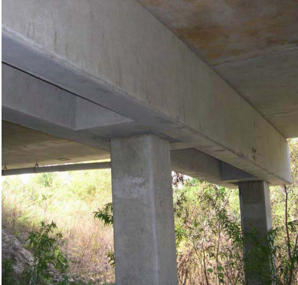
Figure 4-2 Precast Reinforced Concrete Bent Cap [14]
