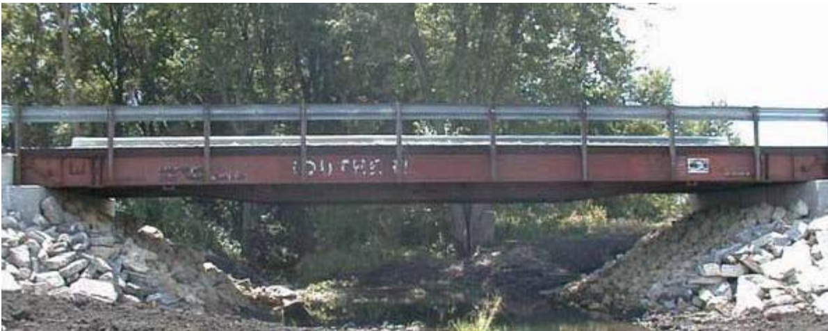
Figure 4-49 Side View of Railroad Flatcar Bridge [57]
