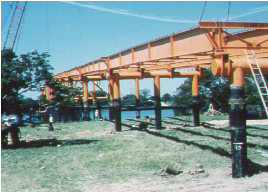
Figure 4-14 Modular Steel Piers [40]
