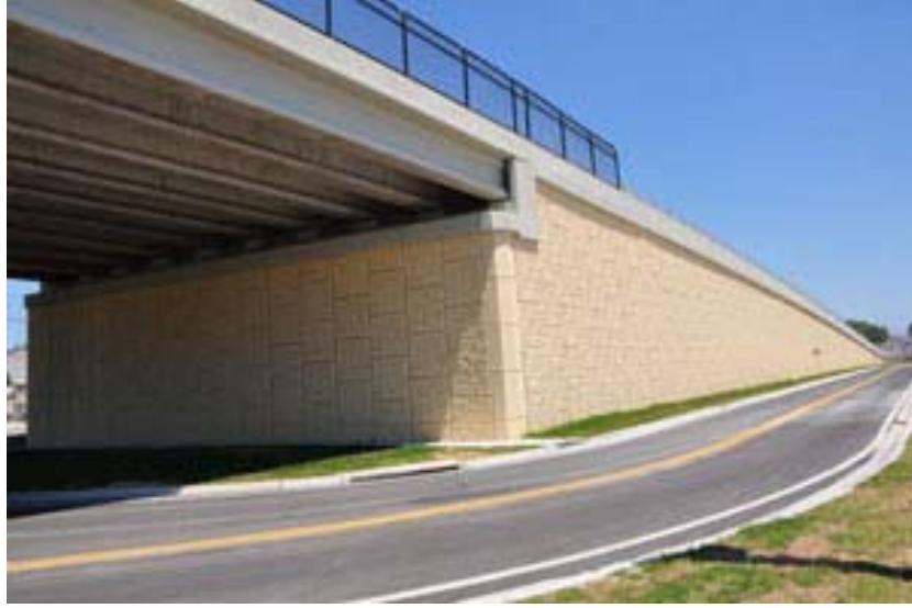
Figure 4-5 Mechanically Stabilized Earth Wing Wall [28]
