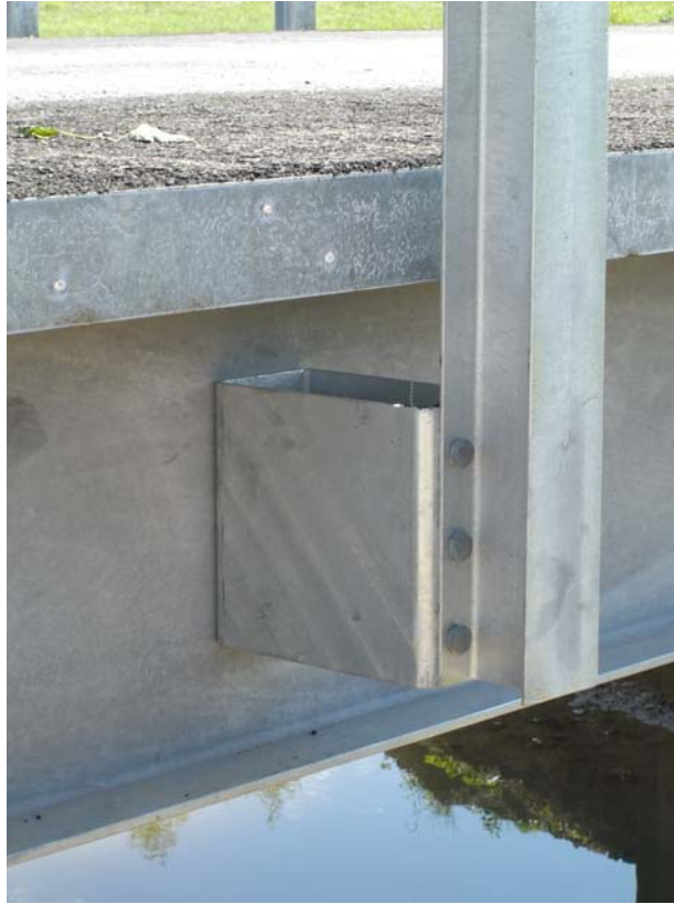
Figure 4-54 Steel Beam Rail Connection (U.S. Bridge Tour)
