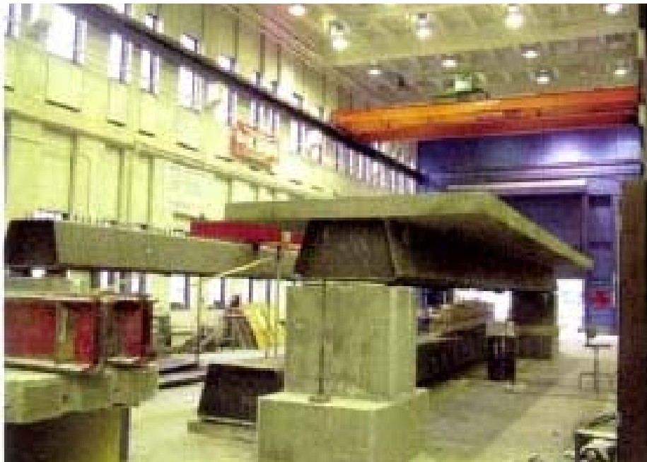
Figure 4-41 Section of Folded Plate Girder Bridge Ready to be Stacked and Shipped [8]
