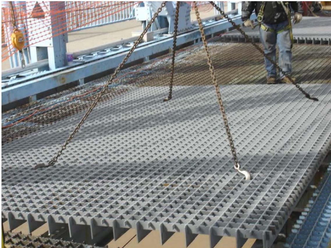
Figure 4-30 Open Grid Decking Being Placed [37]
