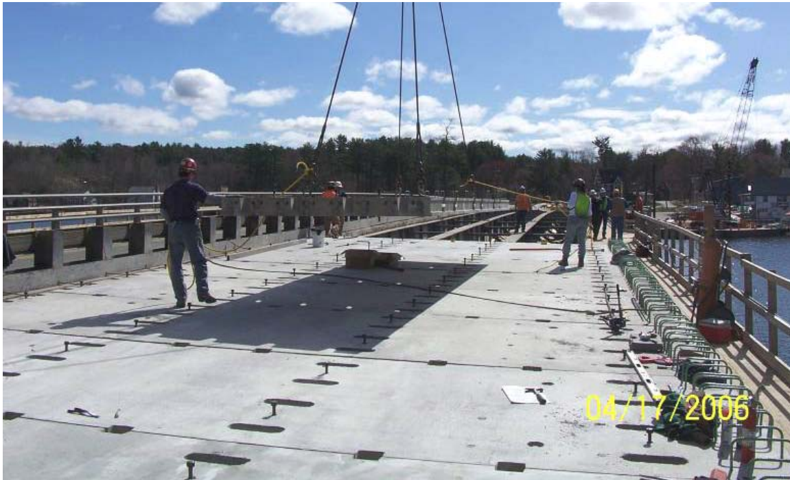
Figure 4-29 Full Depth Precast Deck Panels [14]
