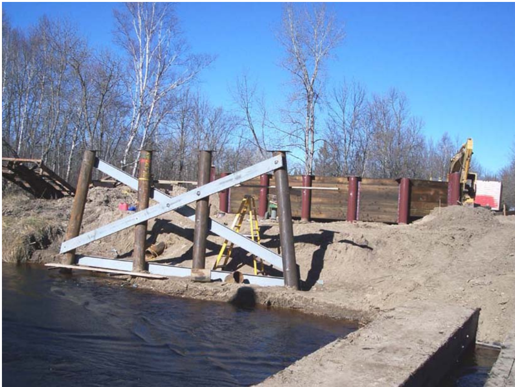
Figure 4-12 Driven Steel Piles for Piers/Abutments [12]
