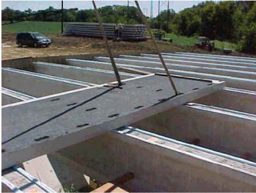
Figure 4-32 FRP Deck Panel Installation [22]
