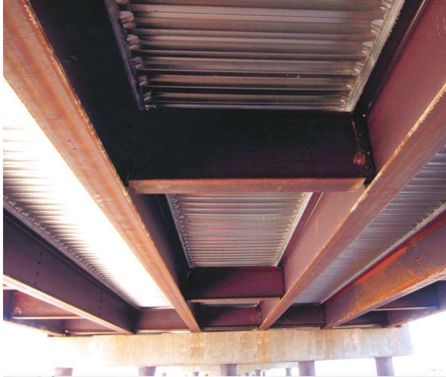
Figure 4-58 Bridge with Steel Diaphragms [31]
